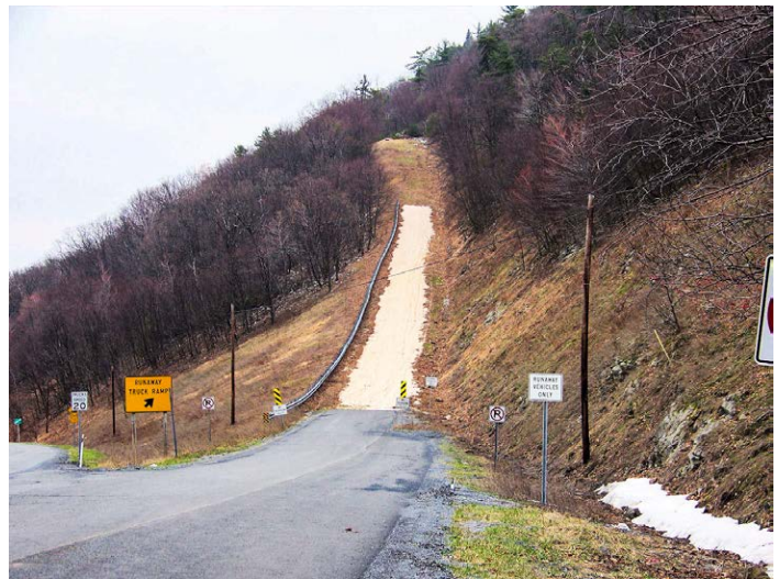
Runaway Truck Ramp, Route 30, PA in the mountains. https://www.publicdomainpictures.net/en/view-image.php?image=6876&picture=runaway-truck-ramp
